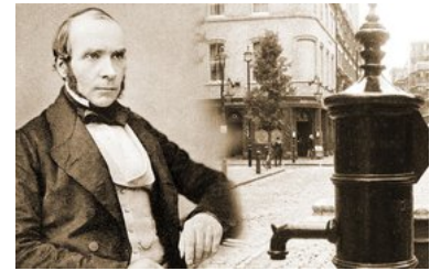
Figure 16.1: DiD is perhaps the oldest quasi-experimental research design. John Snow was a London doctor and is often considered the father of modern epidemiology. [2] is essentially an effort to provide convincing evidence that water is the causal agent for cholera transmission. It presents and discusses multiple pieces of evidence – including a DiD. Source: https://www.micropia.nl/en/discover/microbiology/john-snow/ , accessed 6/7/23.
